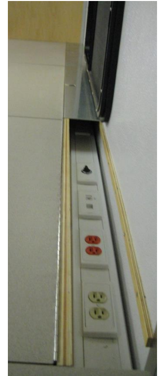
WIREMOLD DUCTING
