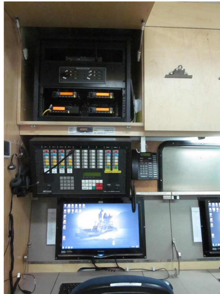
INSTALLATION OF A ZETRON 4010R CONSOLE AND HUGHES 9350 BGAN SATELLITE TRANSCEIVER
